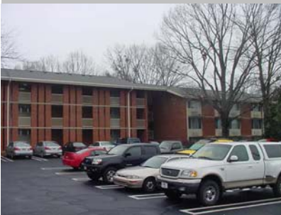
Exterior of Building K, recently remodeled.
